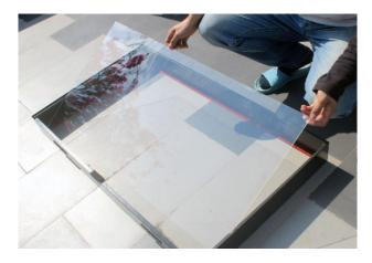
7. Add silicone sealant to the glass/acrylic edge area and all gap area, to ensure it is complete waterproof.
