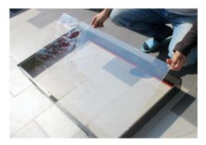
7. Do not remove the back side protective film of acrylic (reduces cleaning issues) then add silicone sealant (Prepare yourself) to the acrylic edge area and all gap area, to ensure it is complete waterproof.
