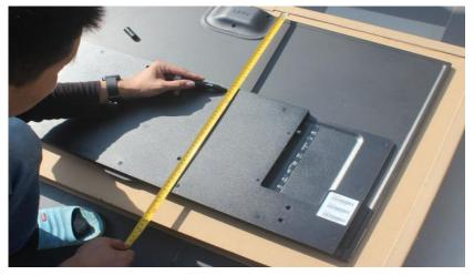
2. Install the Mount arm for the TV, ensure the center point is near the TV middle position.
